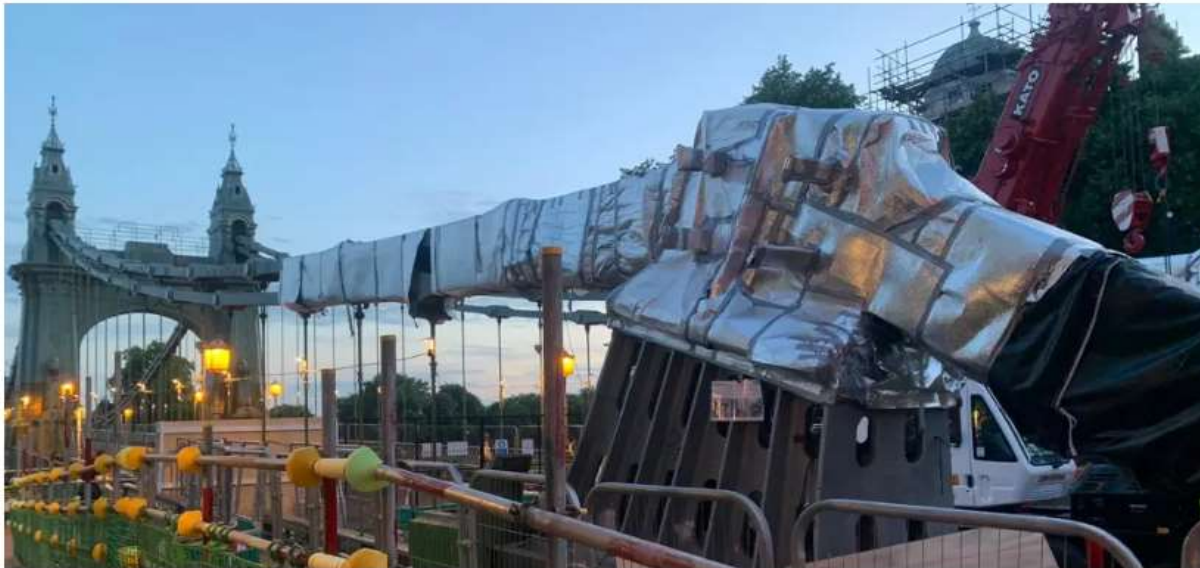
The Hammersmith Bridge wrapped in silver insulation foil in July. Hammersmith & Fulham Council
