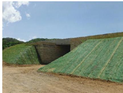
Figure 7. GRS technology used on bridges 1121 and 1122 (Source: PRHTA)
